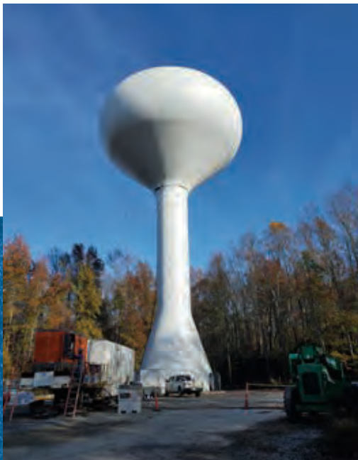
A new elevated storage tank constructed in southern DE.
