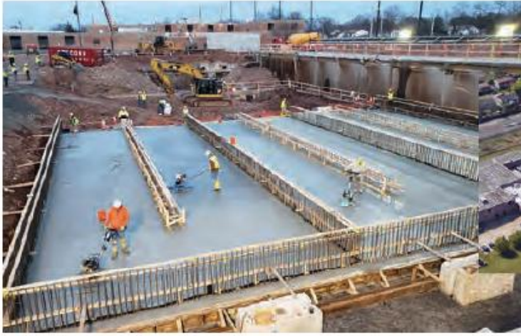
Construction is well underway as workers pour the base slab of the ozone contactors.
